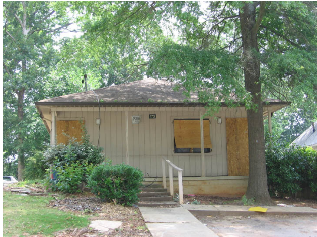
Edgewood Housing Units - Pre-Demolition
