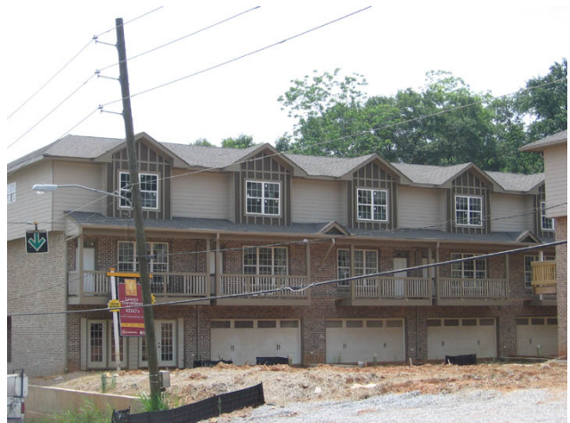
Townhomes Under Construction along Memorial Drive
