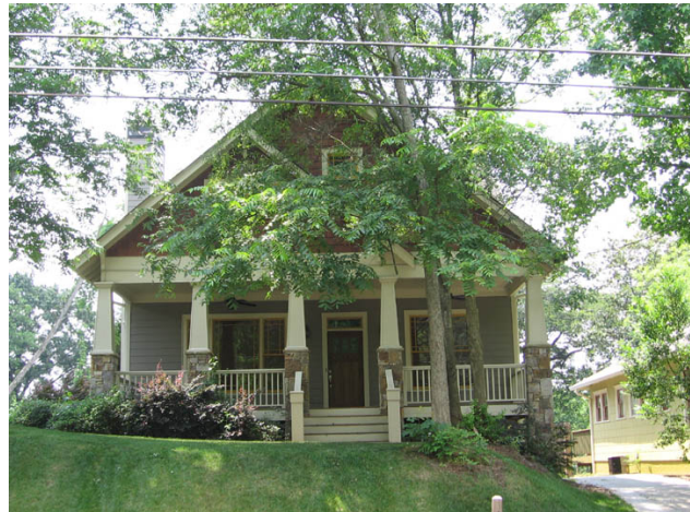
Example of New Infill Housing in Edgewood
