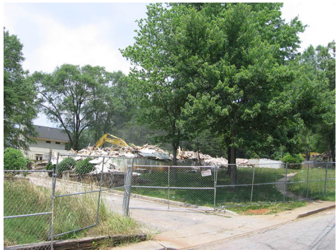
Edgewood Housing Units - Post-Demolition
